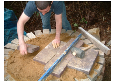
Laying the oven floor
